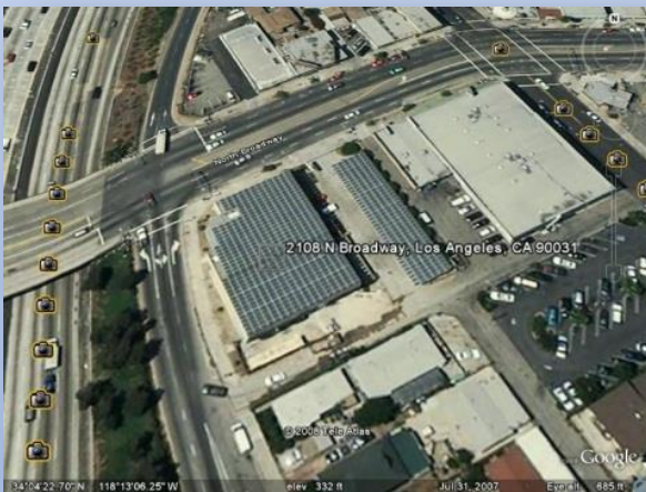
Commercial Building 170KW LA
