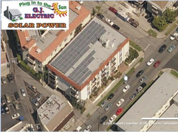
Apartment Building 40KW-Brentwood
